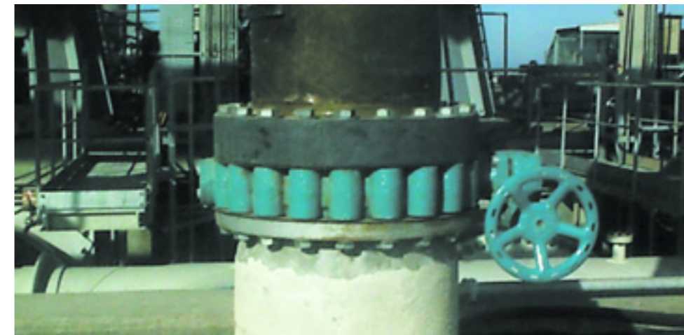
ND 16" ASME / ANSI 150* Lug type, SEA WATER ISOLATION
